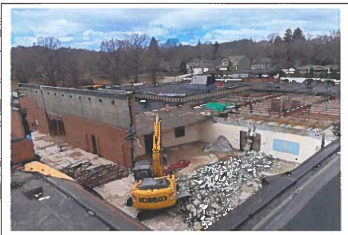
MS & HS Roof & Interior Classroom Demolition
